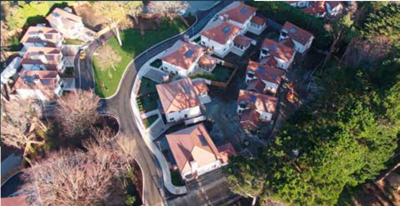
A Brighton Road Foxrock, Dublin 18
