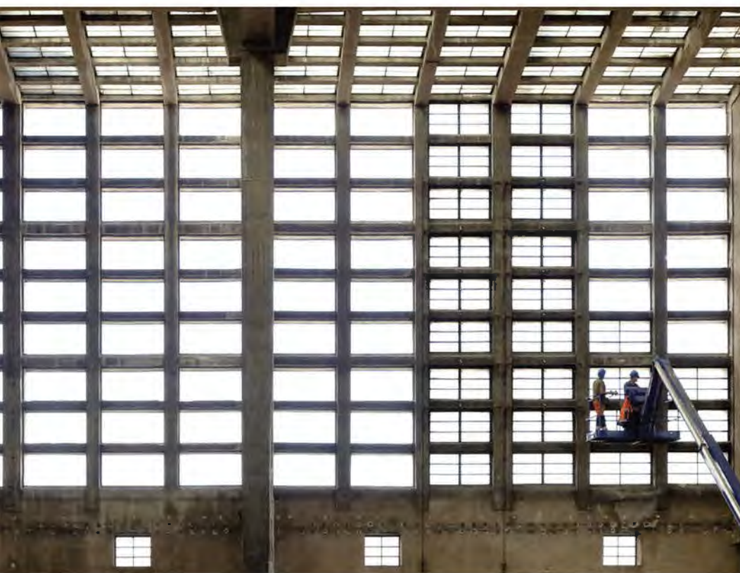
Interior view of the Grossmarkthalle's concrete grid facade. The restoration of the Grossmarkthalle is an important aspect of the construction works. The fundamental appearance of the building will be retained, with its facades and surfaces being restored in line with the preservation order.
